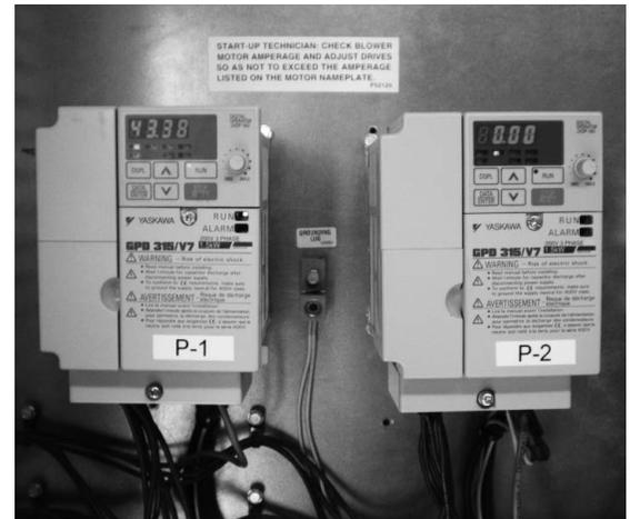
A major benefit of VFDs is their “soft-start” capability that gradually ramps up a motor's operating speed at startup and greatly reduces the stress on components. On typical startup, a constant-speed motor is subject to high torque and electrical surges that can reach up to 10 times the full current load.
