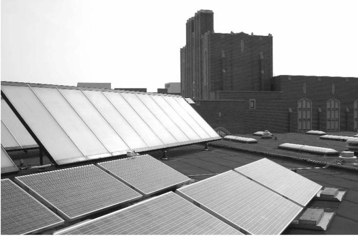
The MGE Foundation worked with Madison's East High School to install the 2.4 kW solar electric system shown in the foreground. Behind it on the left is a solar water heating system. A third solar technology, passive solar skylights, can be seen on the right.
